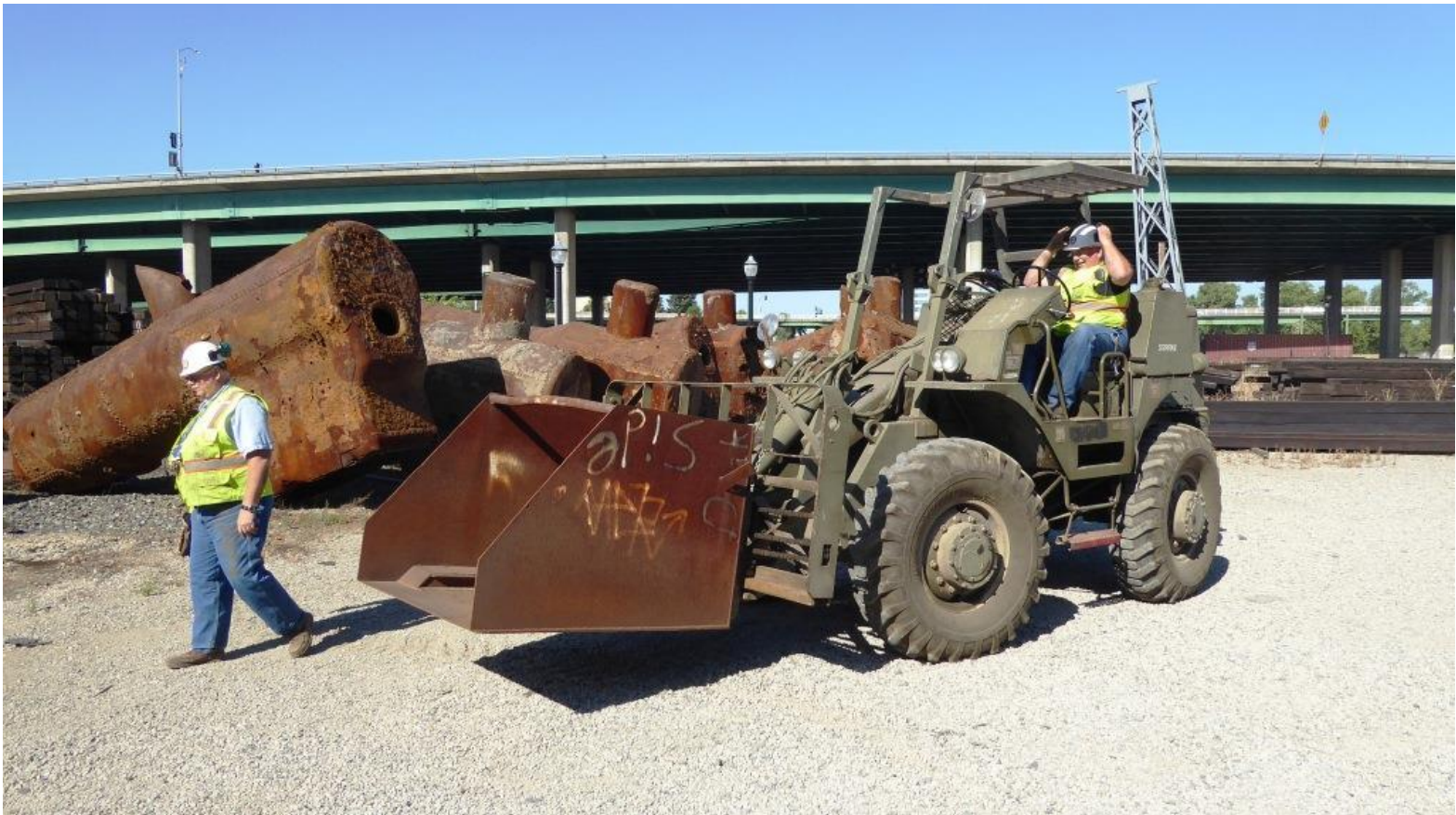
Chris attaches the bucket to GM2's fork and Harry gets ready to join Frank in transporting ballast-rock to the job-site
