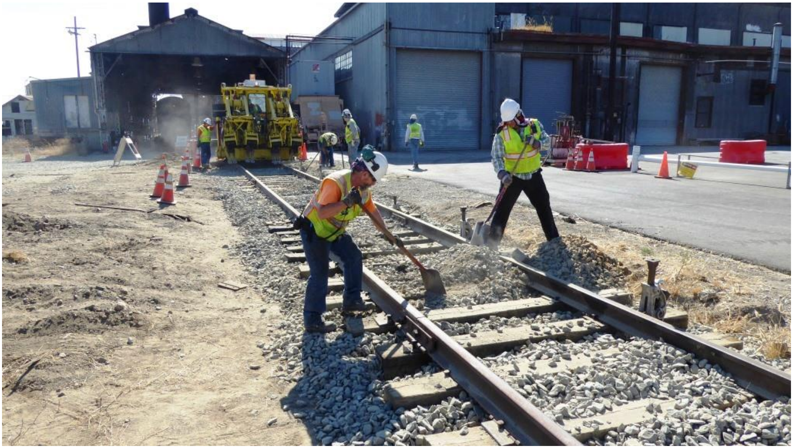
Joe and Jose continue spreading new rock to fill in holes so that there's plenty for the tamper to tamp
