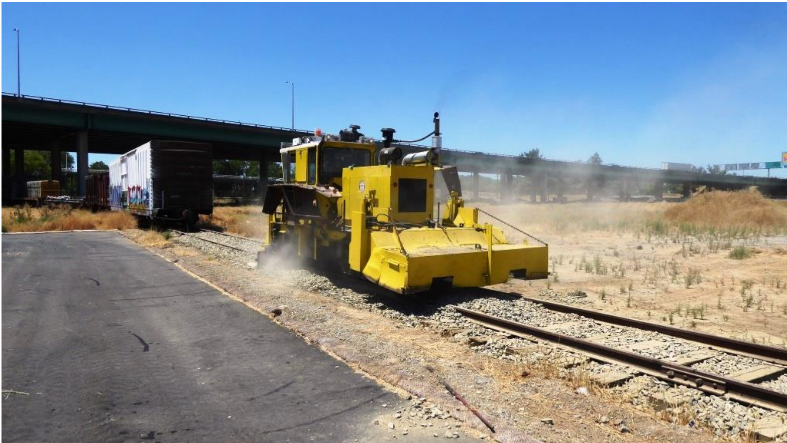
Chris in the regulator starts by pulling rock into the center of the track by running the machine backwards with the plows deployed
