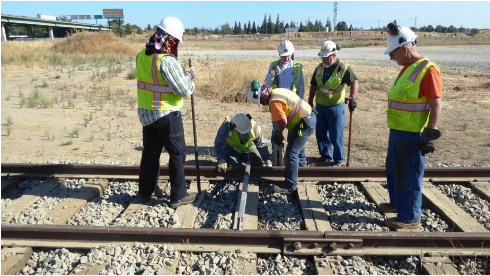
Steve and Joe put on a show as they adjust the jack and read the gauge on the track-level
