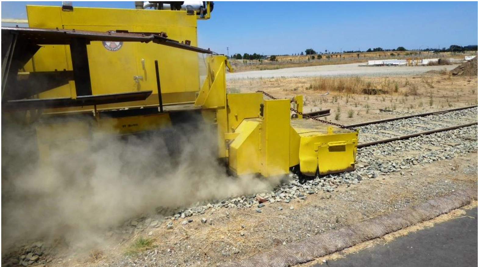
Next, the big spinning broom pushes and compacts the rock between the ties...
