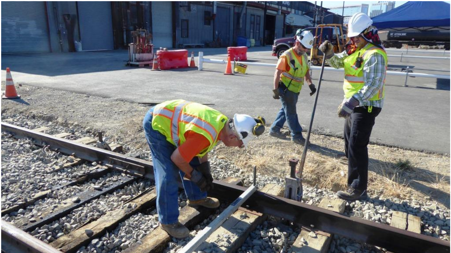
Clem measures the cross-level as Jose cranks on the track-jack
