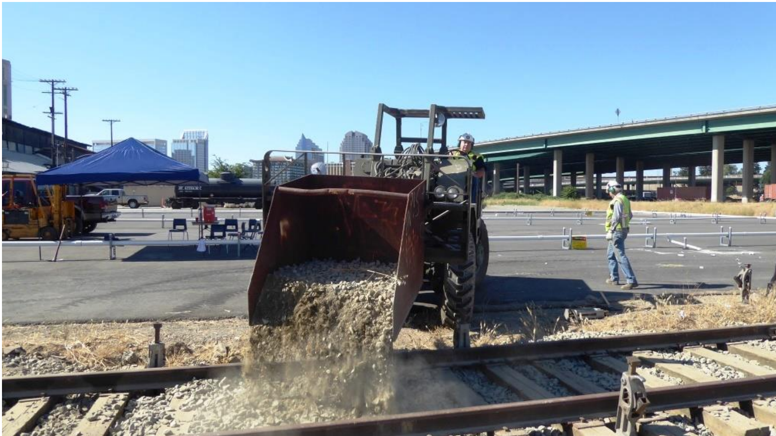
Harry dumps a big scoop of rock onto the track with GM2
